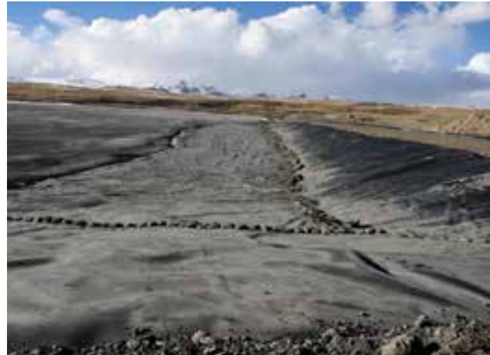
Above; a thick liner is used to prevent seepage into the ground
