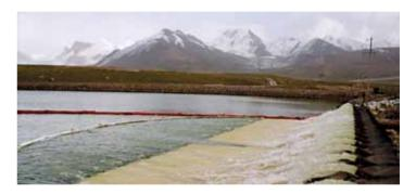
The design of our mill allows us to recycle large quantities of process water. We refer to this as in-mill water recirculation. Annually, we recycle approximately 5.4 million m3 of process water within our mill. During the summer months, when the tailings pond surface and Kumtor River are no longer frozen, we also treat and discharge approximately 5 million m3 of water per year from our Tailings Management Facility.
